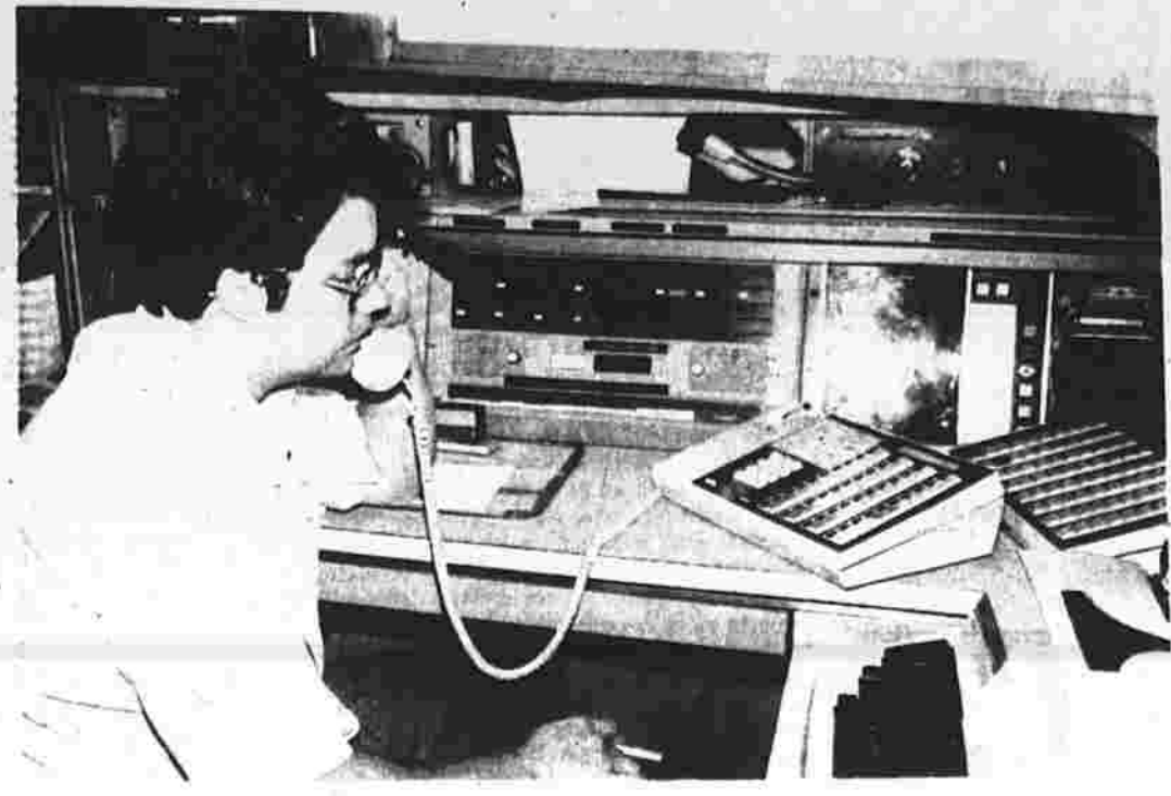
Emergency call Larry Warren, superintendent of communications at the Police Department, answers a call on the 911 emergency line. The 911 line is well-used by Manchester residents for all types of emergencies. (Herald photo by Rosenber)
